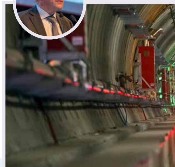
LIEFKENSHOEK RAILWAY TUNNEL Antwerp, Belgium
