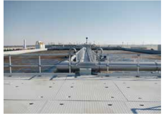
RUWAIS SEWAGE TREATMENT PLANT Al Ruwais, UAE
